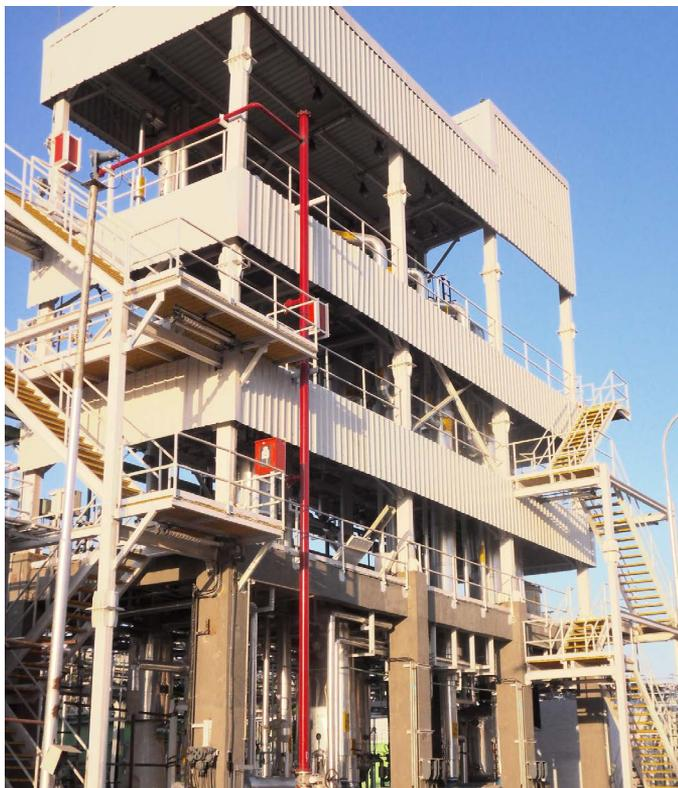
Secondary Treatment by Membrane Bio-reactor (MBR) process: In secondary treatment, a composite unit consisting of aeration and membrane filtration (membrane bio-reactor) is provided for bio-logical treatment. The unit is designed to meet pollution control norms and / or to feed treated effluent to reverse osmosis unit.
